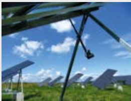
Former landfill site with 54 DEGER TOPtrackers®, Germany
