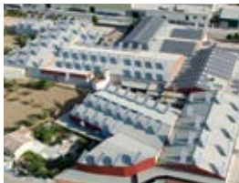
Roof system with 120 DEGER TOPtracker®, Spain
